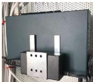
The POF cables are parked in the multimedia distribution cabinet. For example with Wago clamps. To activate the optical fibre connections, the parked cables are connected to an active POF network component eg. POF Switch or POF media converter.
