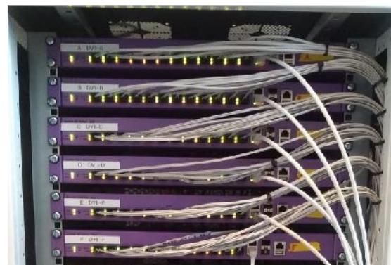
In this network rack some POF 12+4 port switches are connected together and so they provide many network connections in the different rooms of this hotel.
