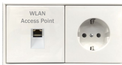
WiFi access points can be integrated into the electrical installation.
