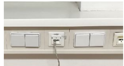
IN SURFACE CABLE CHANNEL
